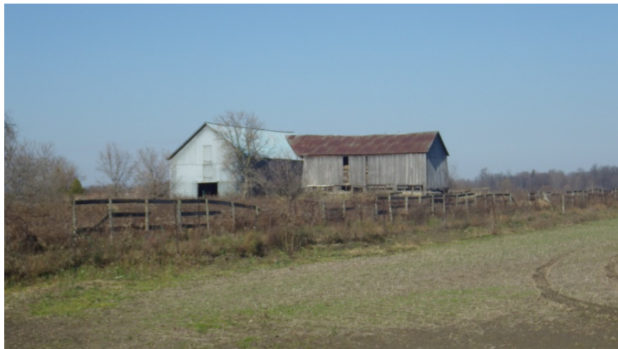
Plate 4: 6771 Young Street, barn, looking north
