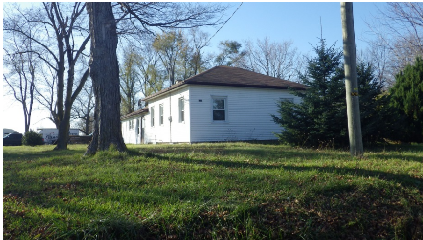
Plate 5: 6736 Regional Road 20, looking south
