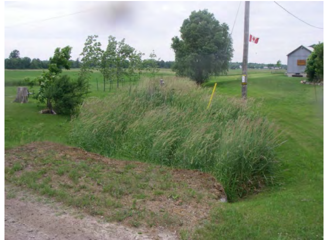
Photo 16: Station R11T081-A – Black Ash Creek (Summer 2012) - Facing upstream (northwest) off of Concession 4, showing channel of Reed Canary Grass adjacent to manicured lawn.
