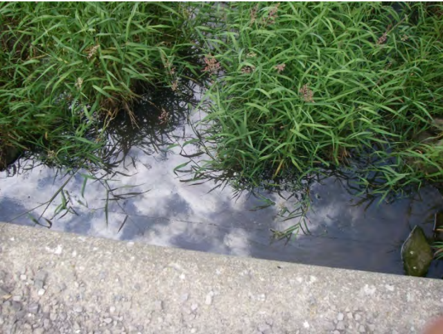
Photo 21: Station R11T097-2 – Black Ash Creek (Summer 2012) - Off of Silver Street, showing water in channel by culvert.
