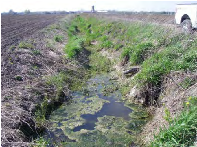
Photo 3: Station R11T091-1 – Unnamed Tributary to Upper Welland River (Summer 2012) - Facing downstream (southeast) east of Gore Road, showing channel overview next to farm path.
