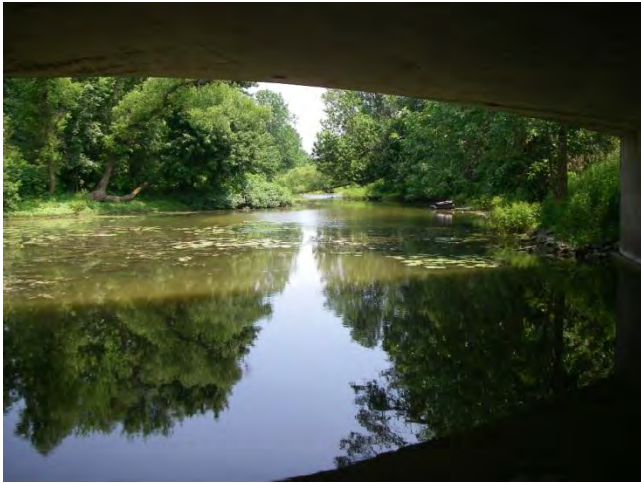
Photo 7 Station 11-2 – Twenty Mile Creek (Summer 2012) - Facing downstream (southeast) from South Grimsby Road 6, showing channel from bridge.
