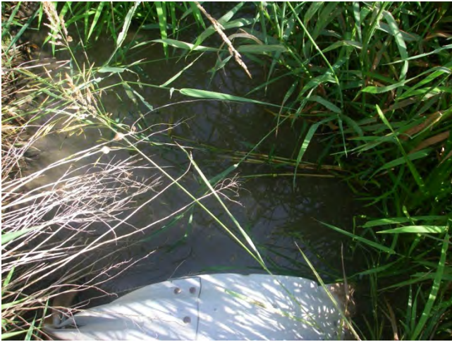
Photo 7 Station 54-1 – Sixteen Mile Creek (Summer 2012) – Showing culvert and pooling water.
