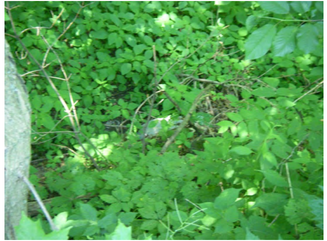
Photo 14 Station 3-2– Beamsville Creek (Summer 2012) - Facing west from Mountainview Road, showing sunken culvert.
