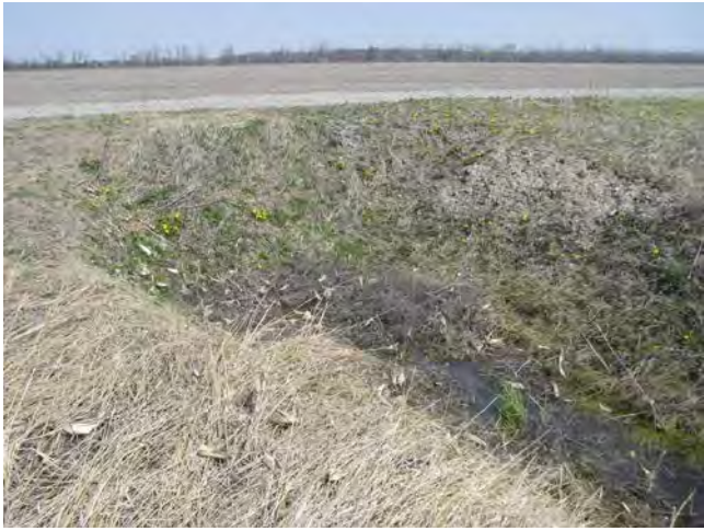
Photo 25: Station R11T045-3—Broad Creek Drain (Summer 2012) – Facing upstream (north) south of Canal Bank Road, showing shallow channel on edge of agricultural field.
