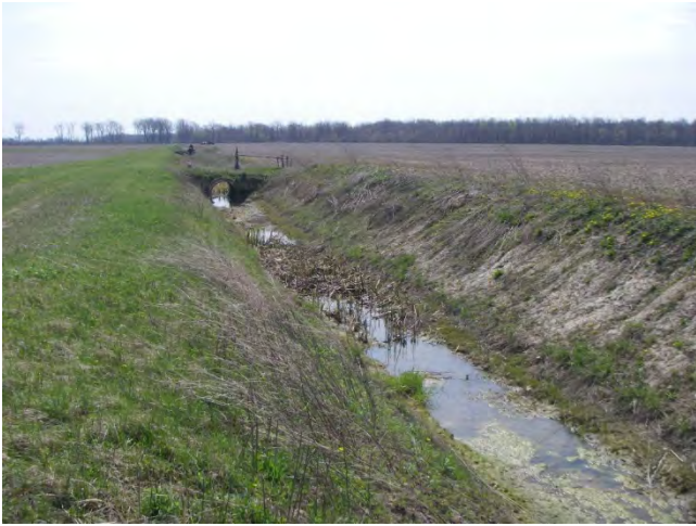
Photo 1: Station R11T016-1 – Low Banks Drain (Summer 2012) - Facing upstream (south) south of Canal Bank Road, showing channel and adjacent fields.
