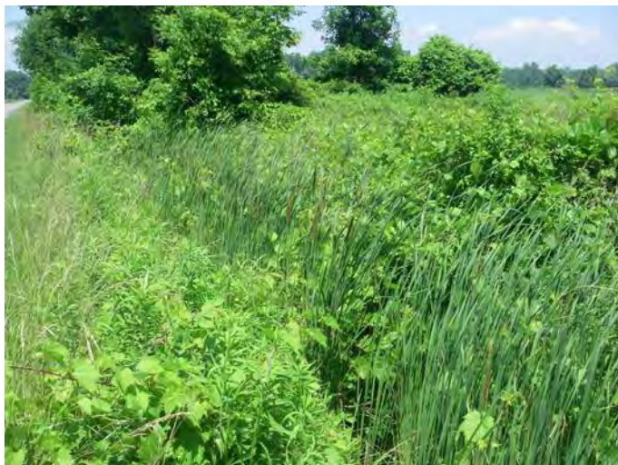
Photo 1: Station 77-1 – Tweed Drain (Summer 2012) - Facing upstream (northeast) from Bird Road, showing channel overview.
