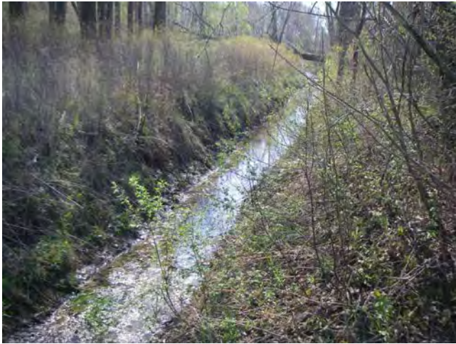
Photo 25: Station R11T084-1 – East Kelly Drain (Summer 2012) - Facing downstream (east) south of Jenny Jump Road, showing channel overview.
