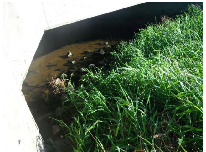
Photo 42: Station SGR3-1 – Spring Creek (Summer 2012) – From South Grimsby Road 3, showing channel and substrate.
