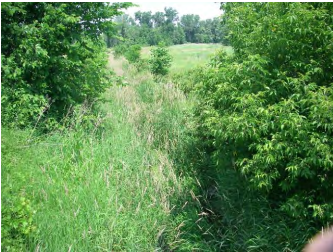
Photo 17: Station 66-2 – Big Forks Creek (Summer 2012) - Facing downstream (northeast) from Wellandport Road, showing channel overview.
