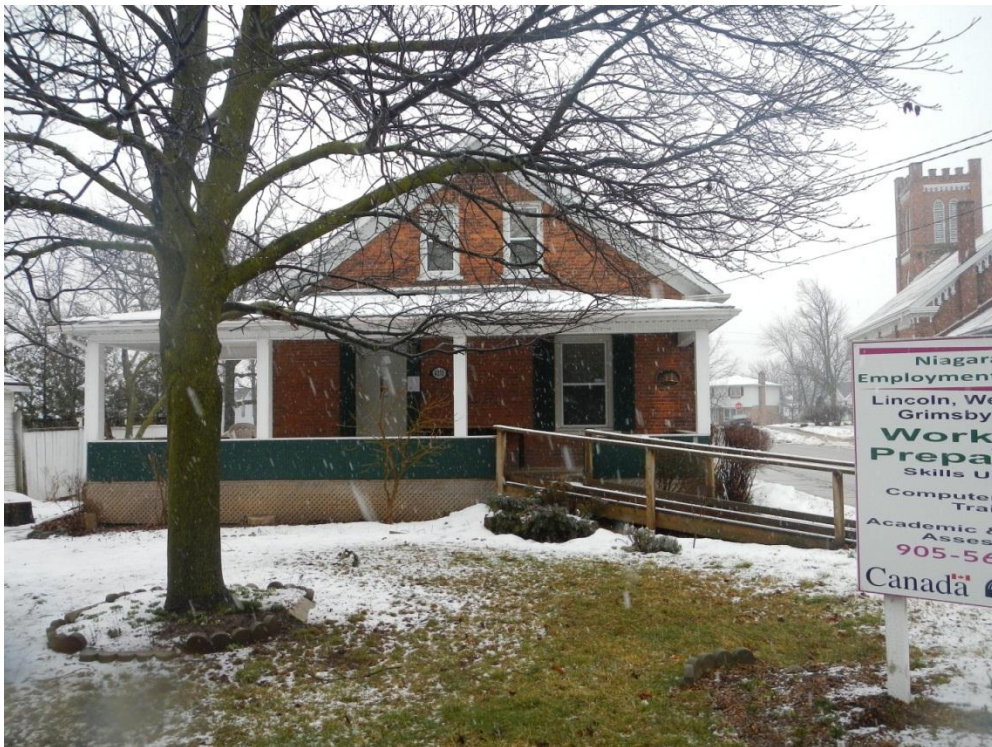
Photo 28: 4721 Queen Street, Beamsville, The Howard House, front elevation
