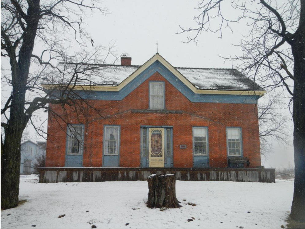
Photo 25: 5499 Philp Road, Marlatt Farmstead, front elevation
