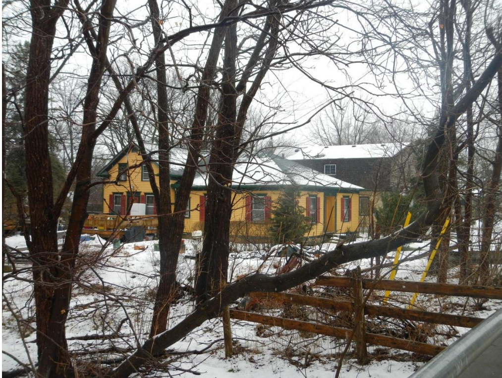
Photo 21: 205 Canborough Street, side elevation
