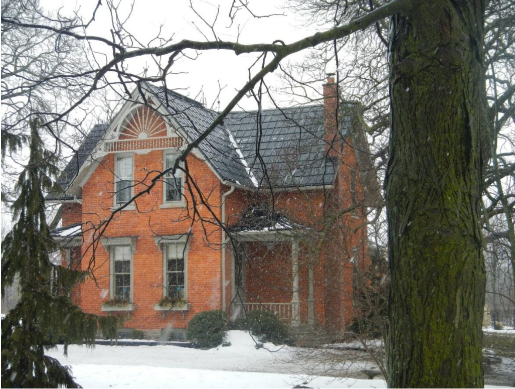
Photo 14: 2663 Moote Road, Former Moot House
