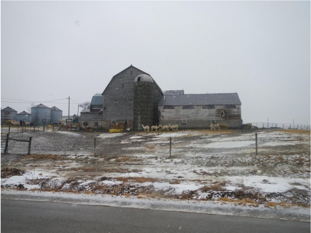
Photo 8: 1639 Rosedene Road, Comfort Barn front elevation
