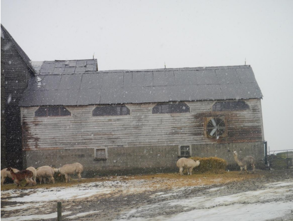
Photo 12: 1639 Rosedene Road, Comfort Barn, south section with louvers
