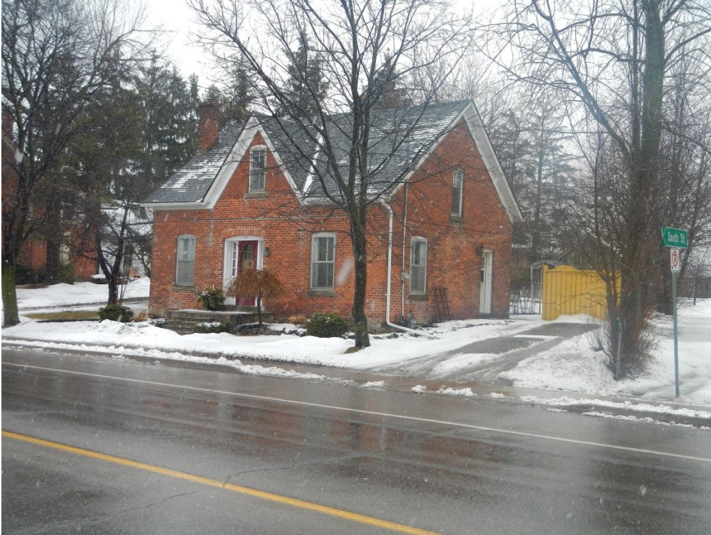
Photo 18: 139 St. Catherines Street, Smithville, side elevation
