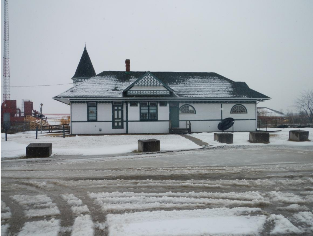
Photo 23: Smithville Train Station
