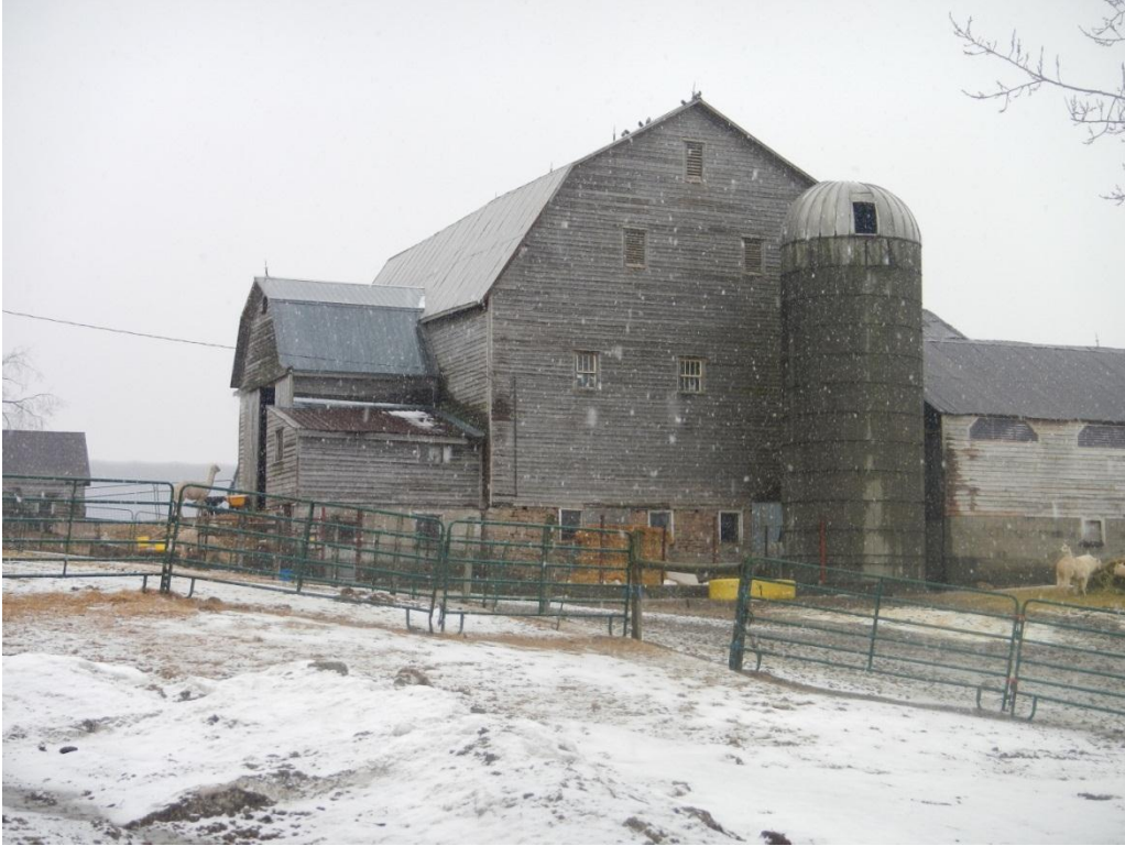
Photo 9: 1639 Rosedene Road, Comfort Barn, north end
