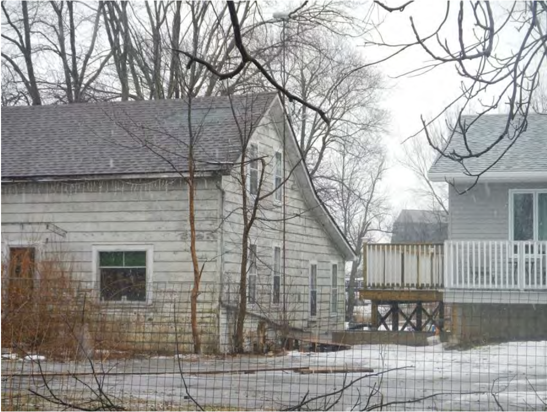
Photo 122: 664 Marshagan Road, south side
