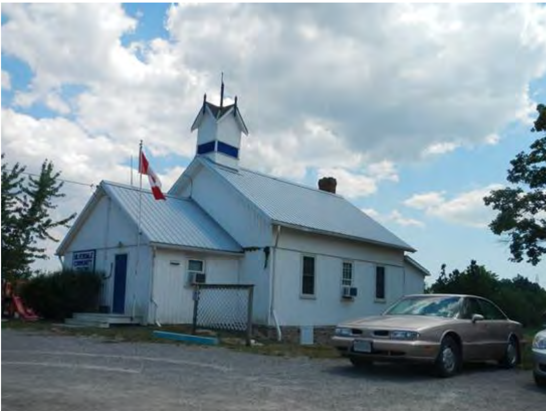
Photo 34: Silverdale Community Centre
