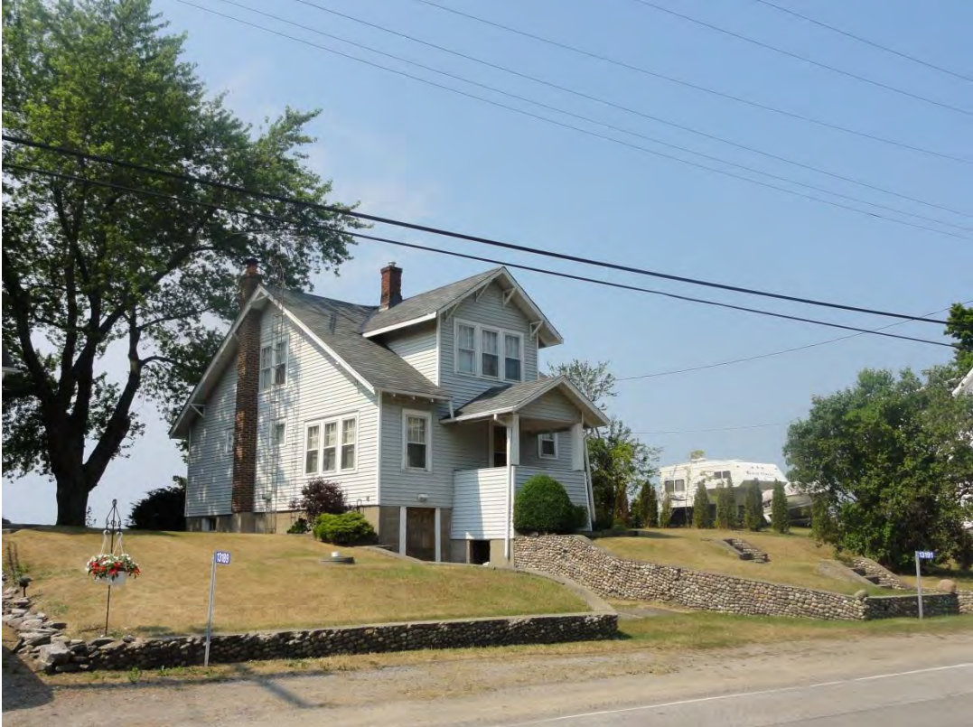
Photo 140: Lowbanks Streetscape Cultural Heritage Landscape
