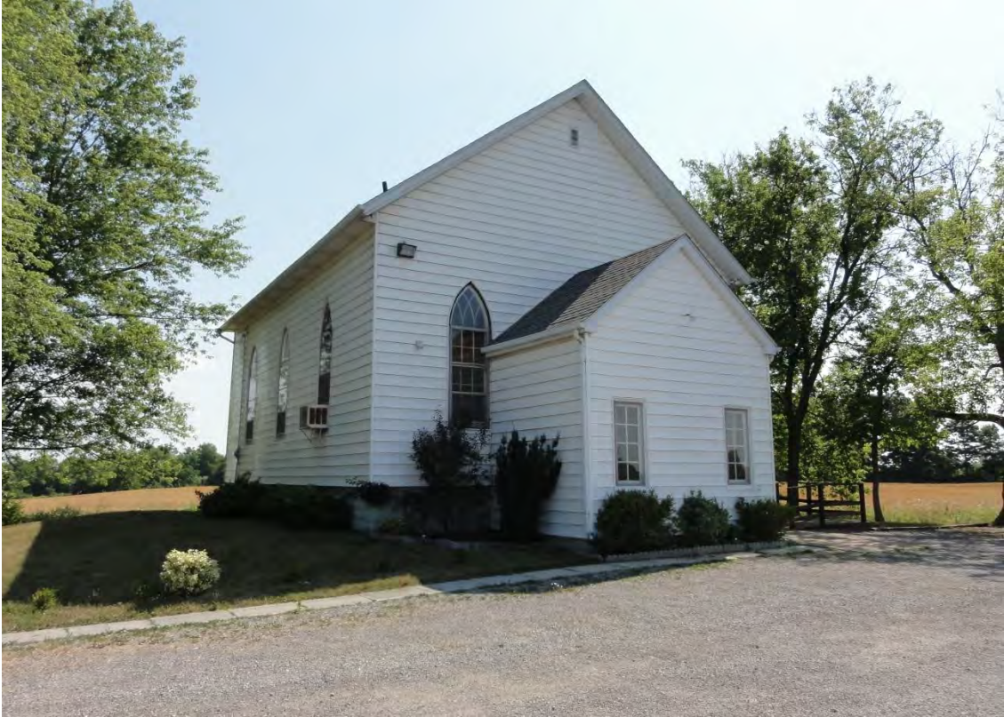
Photo 80: Wellandport Church of Christ
