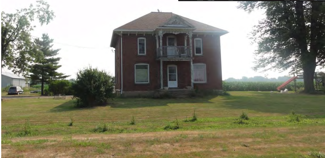
Photo 124: 753 Inman Road, inset showing porch pediment detailing
