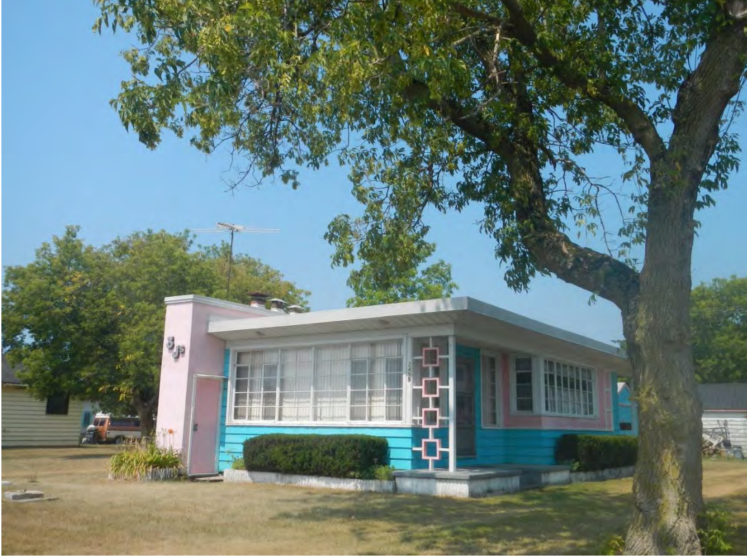
Photo 143: Lowbanks Streetscape Cultural Heritage Landscape
