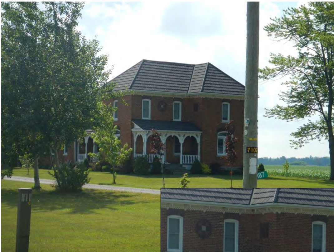
Photo 70: 1187 Heaslip Road, inset showing brick detailing
