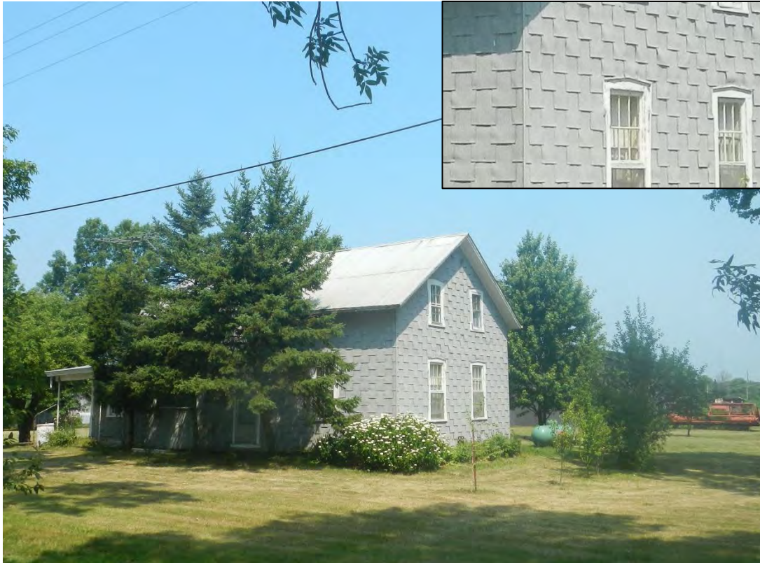
Photo 128: 2307 North Shore Drive, inset showing exterior cladding
