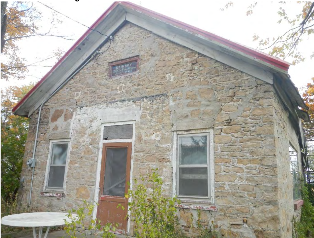
Photo 154: Former Schoolhouse (3263 South Grimsby Road 3)
