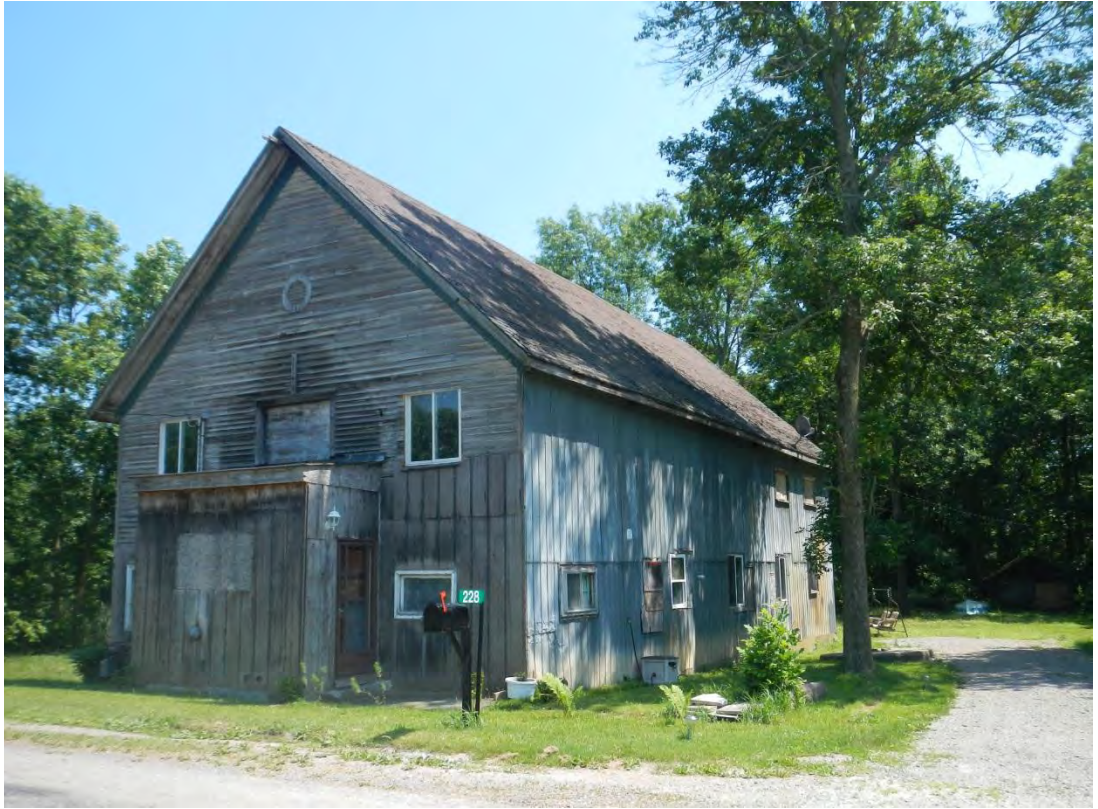
Photo 126: 228 Feeder Canal Road
