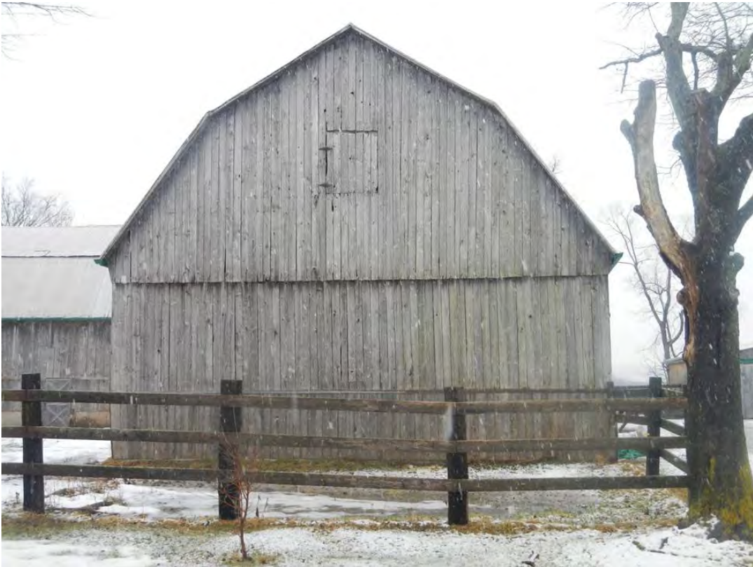
Photo 116: 214 Gore A Road, gambrel roof barn section facing road
