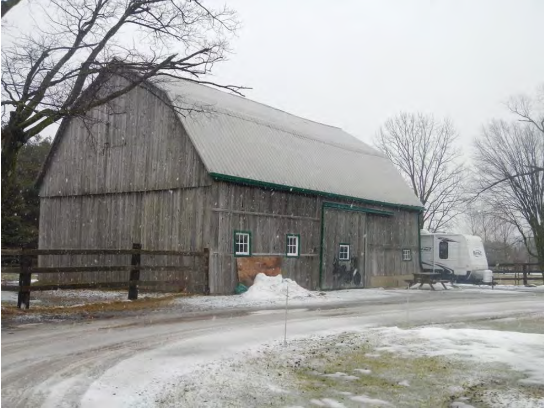
Photo 115: 214 Gore A Road, south west side of barn
