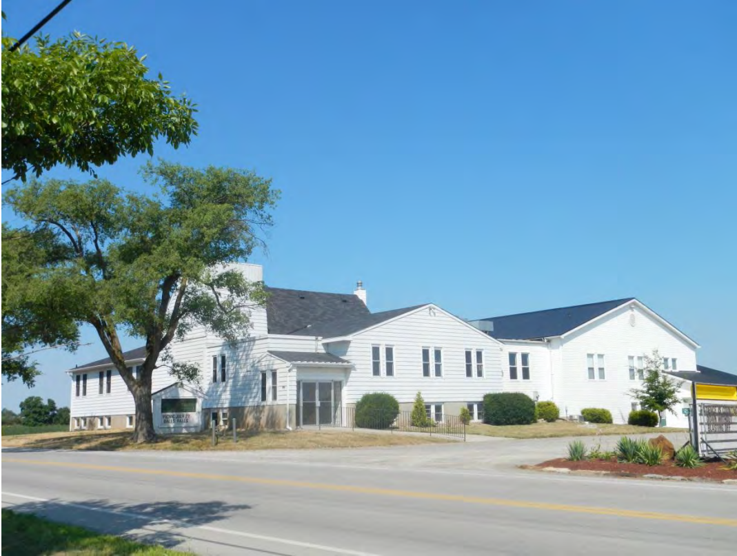
Photo 47: St. Ann's Community Church and Cemetery, showing rear additions to church
