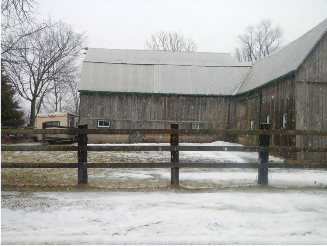
Photo 117: 214 Gore A Road, gambrel roofed barn section parallel to road
