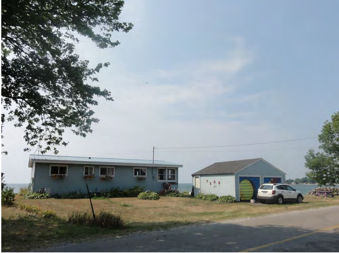
Photo 141: Lowbanks Streetscape Cultural Heritage Landscape
