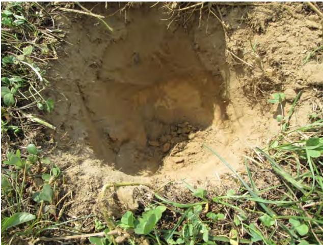
Photo 95: Detail of test pit from Tie-in.
