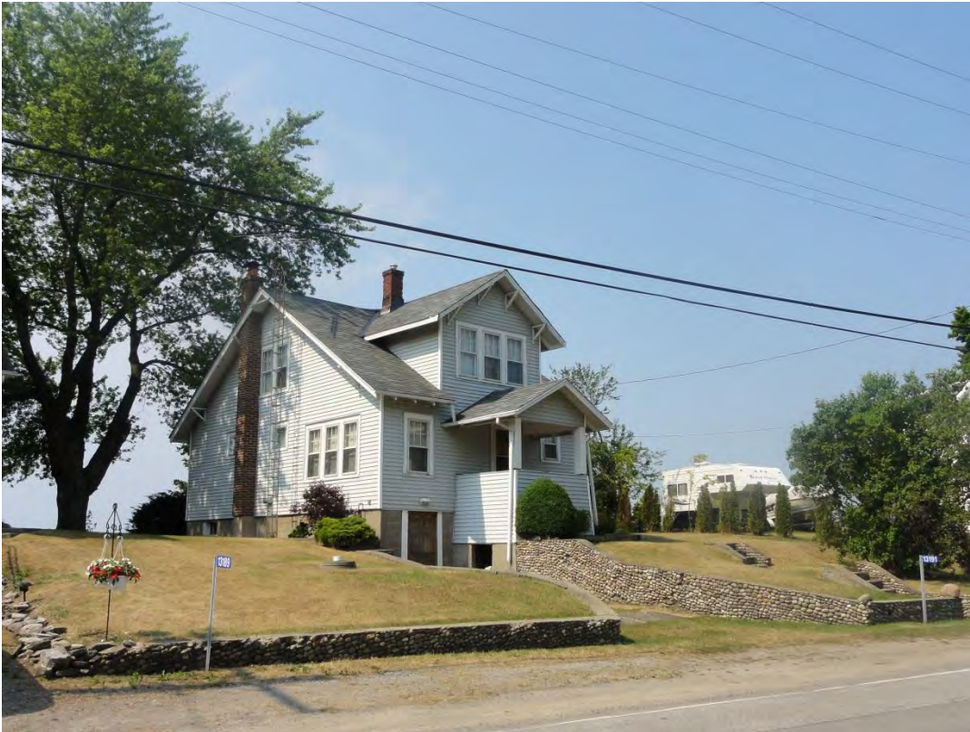
Photo 140: Lowbanks Streetscape Cultural Heritage Landscape
