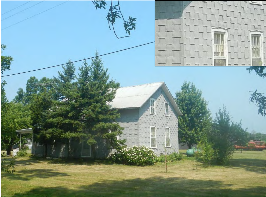
Photo 128: 2307 North Shore Drive, inset showing exterior cladding
