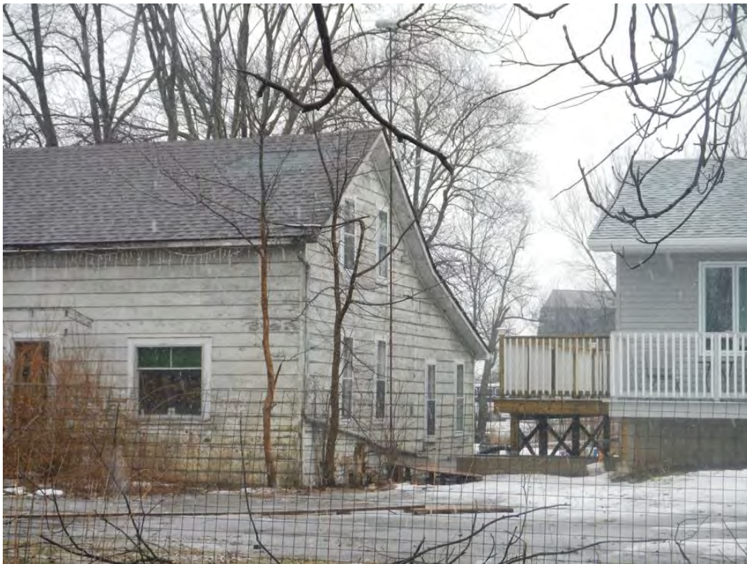
Photo 122: 664 Marshagan Road, south side
