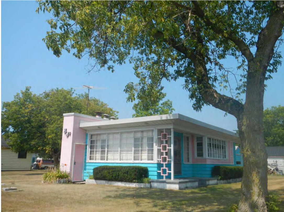
Photo 143: Lowbanks Streetscape Cultural Heritage Landscape
