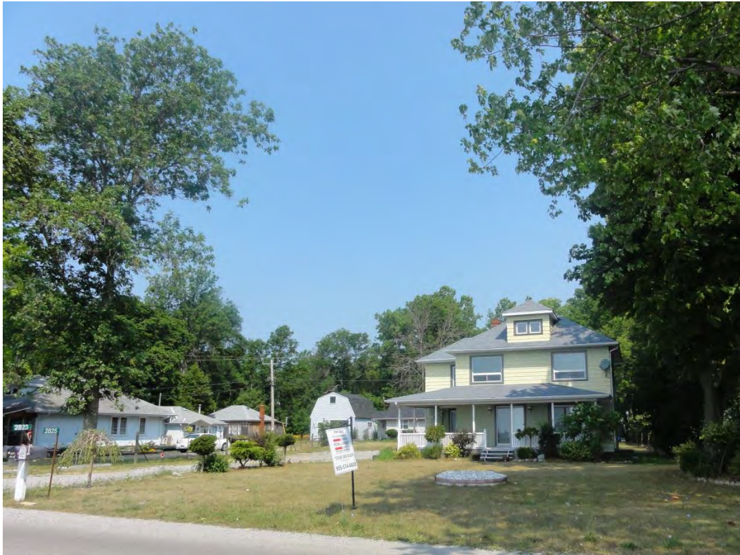
Photo 142: Lowbanks Streetscape Cultural Heritage Landscape
