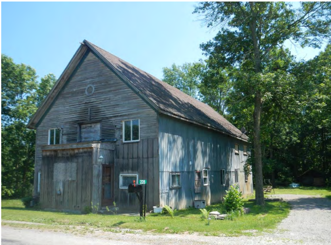
Photo 126: 228 Feeder Canal Road
