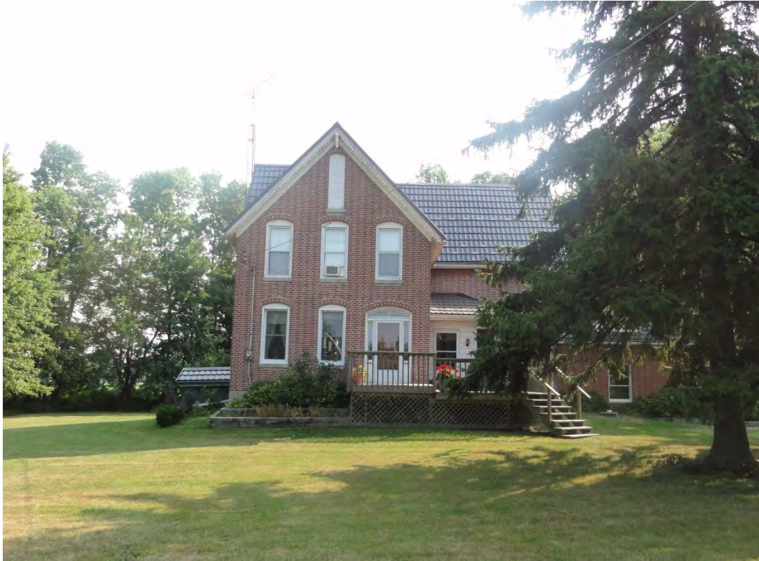
Photo 125: 928 Canal Bank Road
