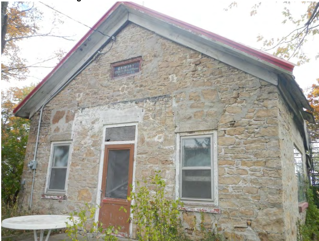
Photo 154: Former Schoolhouse (3263 South Grimsby Road 3)
