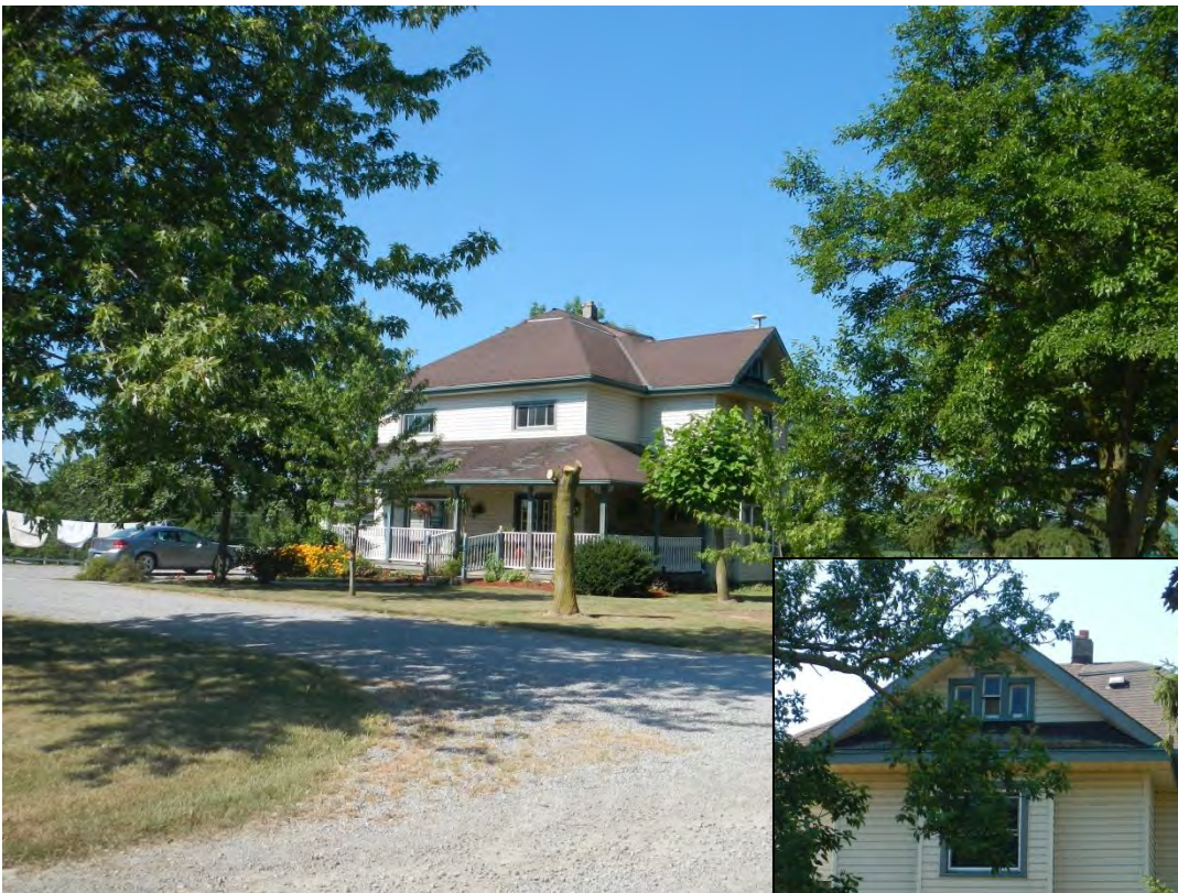
Photo 56: 7092 South Chippewa Road, inset showing attic design
