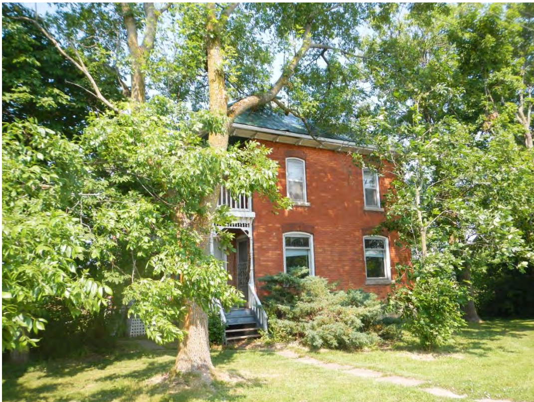
Photo 8: 1500 Caistor Gainsborough Townline Road
