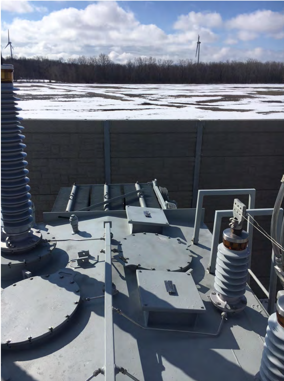
Picture 1 : South Substation Walls, Looking South
