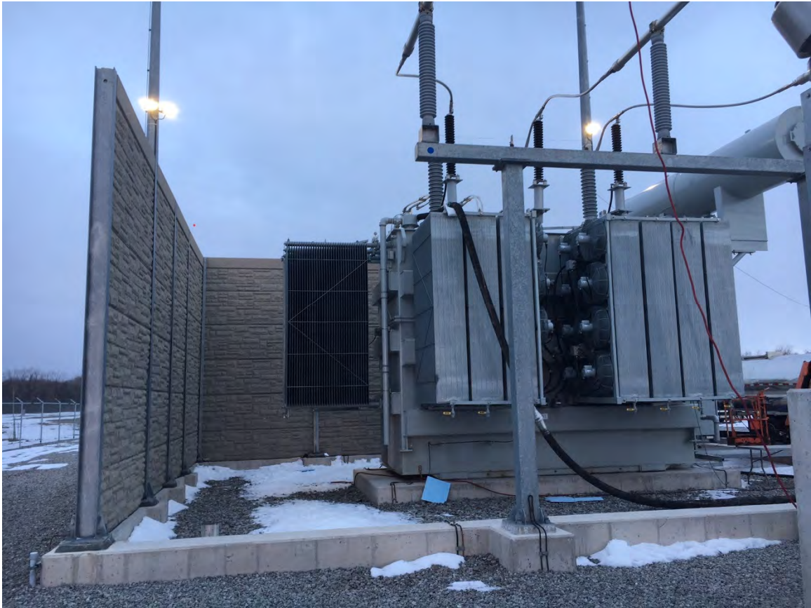
Picture 2 : South Substation Walls, Looking West
