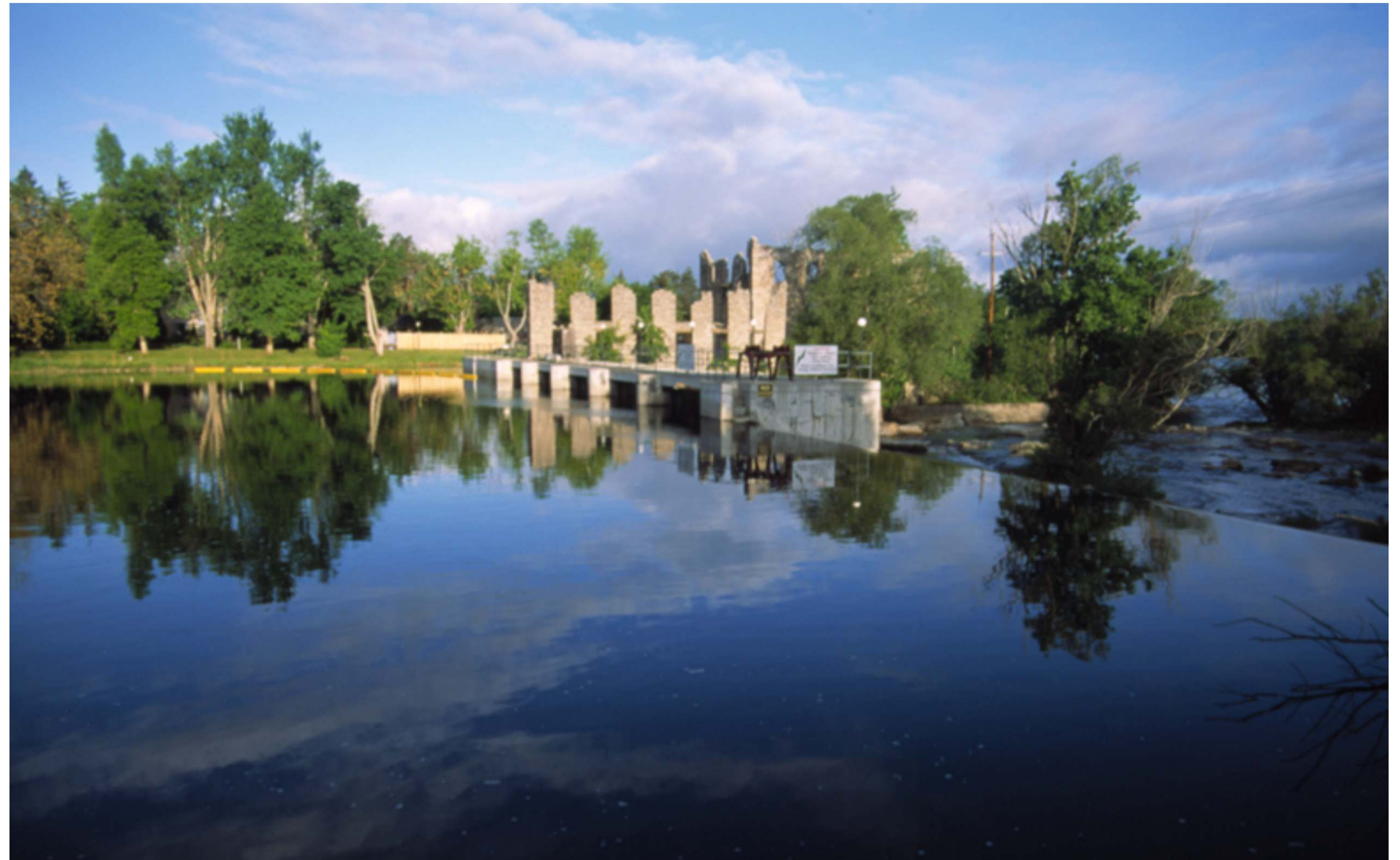
1.4 MW Appleton Hydroelectric Plant, Ontario
