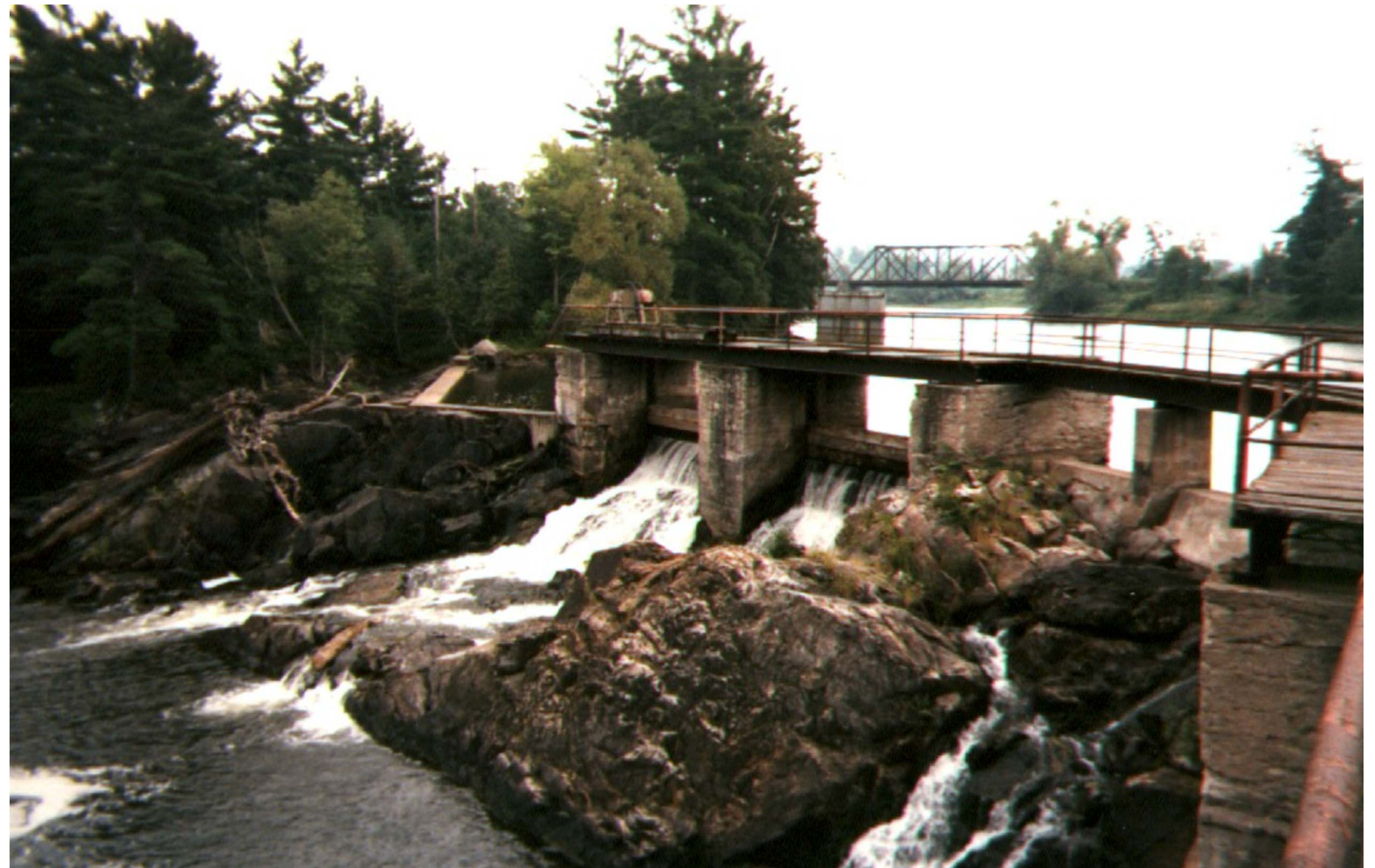
1.6 MW Galetta Hydroelectric Plant, Ontario
