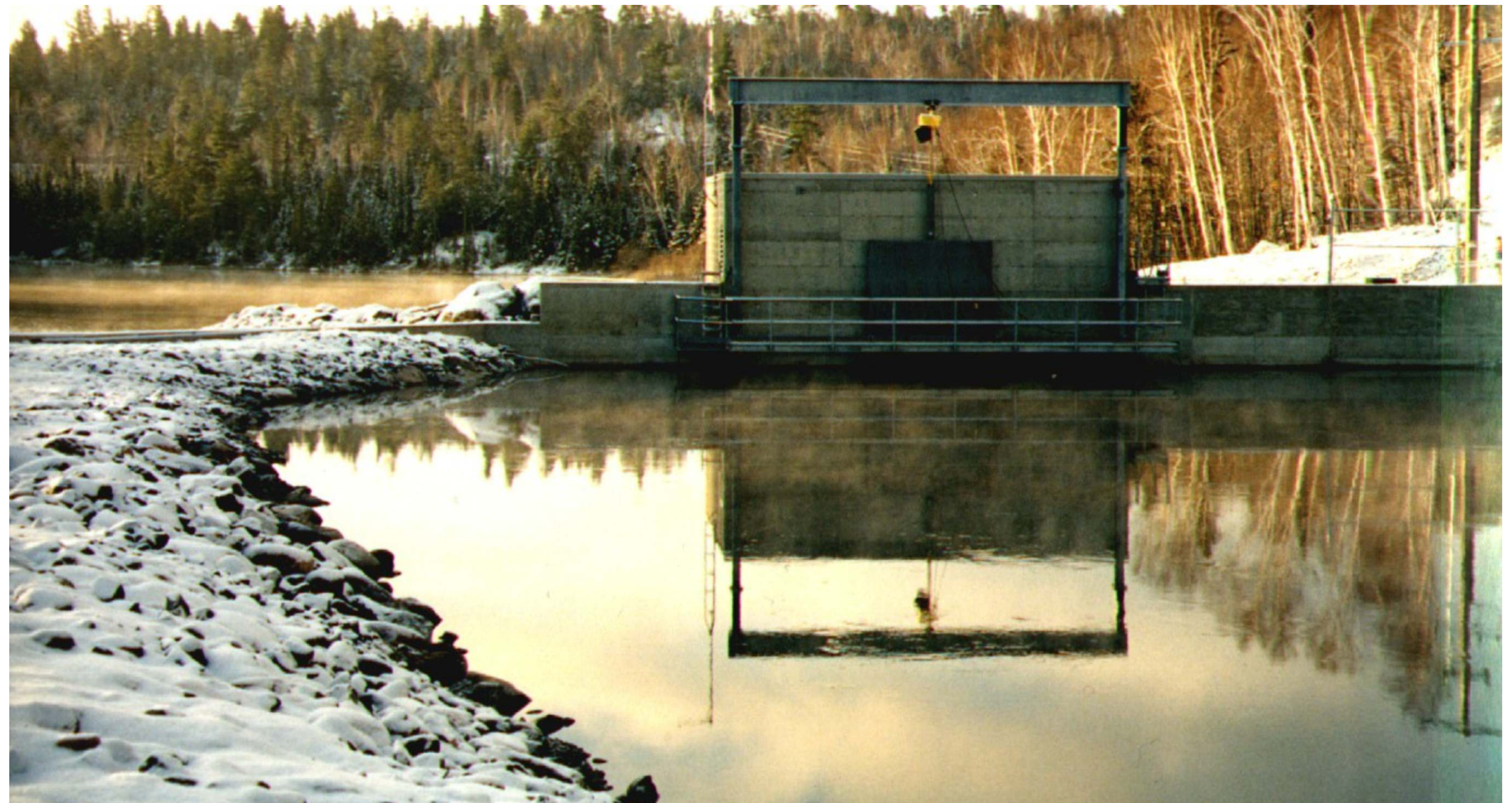
1.3 MW Moose Rapids Hydroelectric Plant, Ontario
