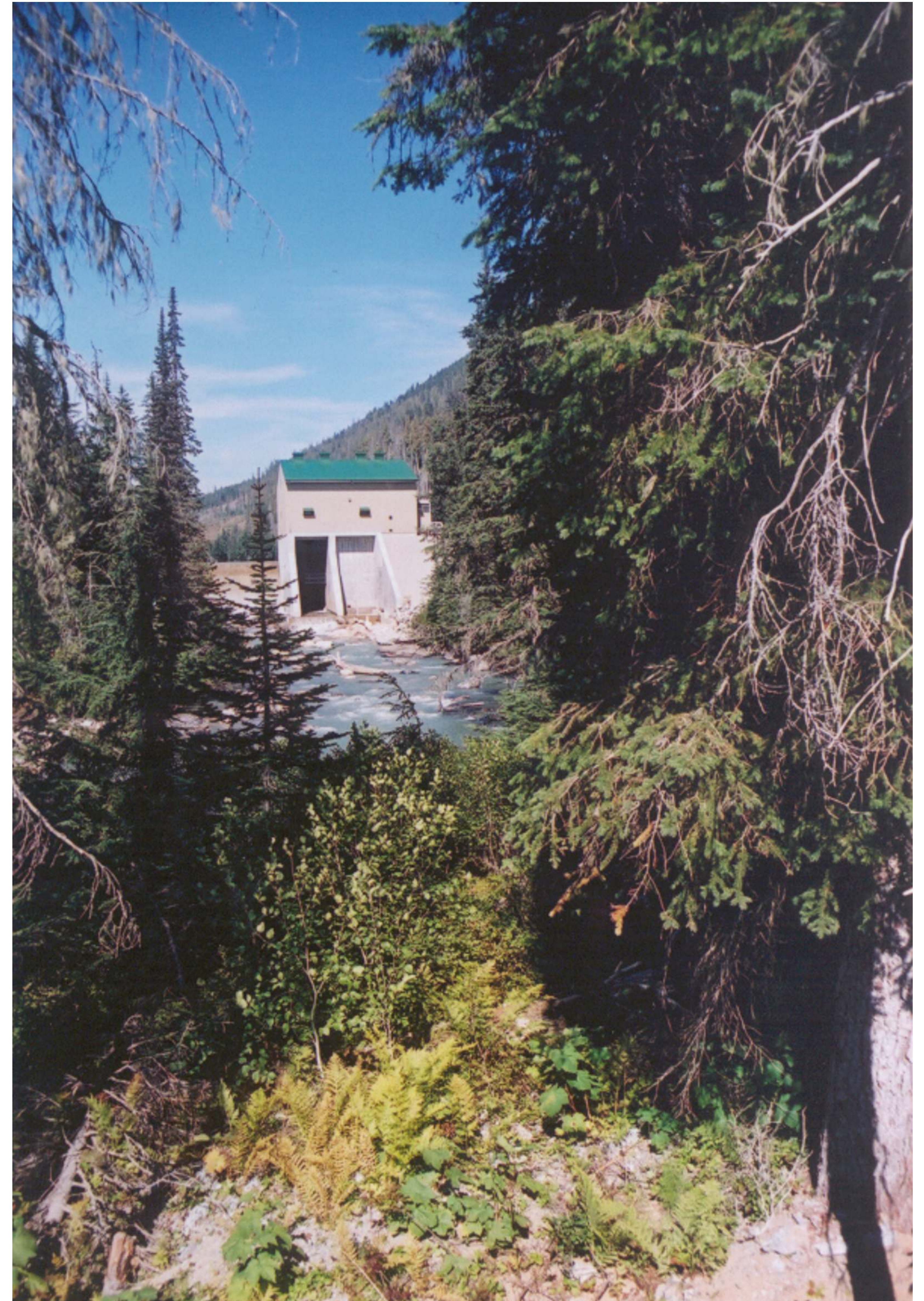
45 MW Pingston Hydroelectric Plant, British Columbia
